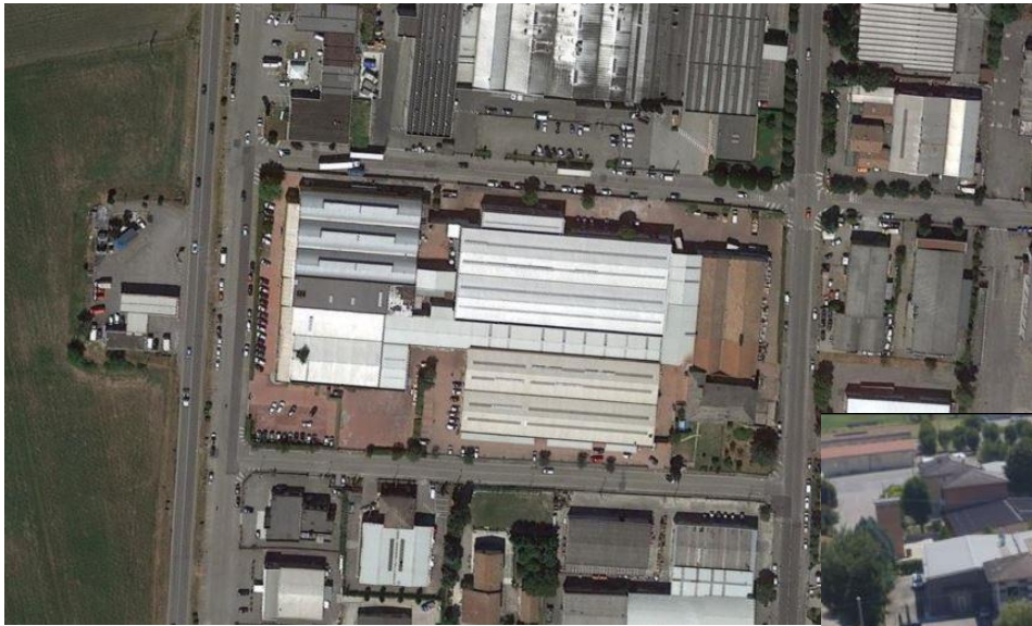
V. Fermi factory roof before photovoltaic plants installation
