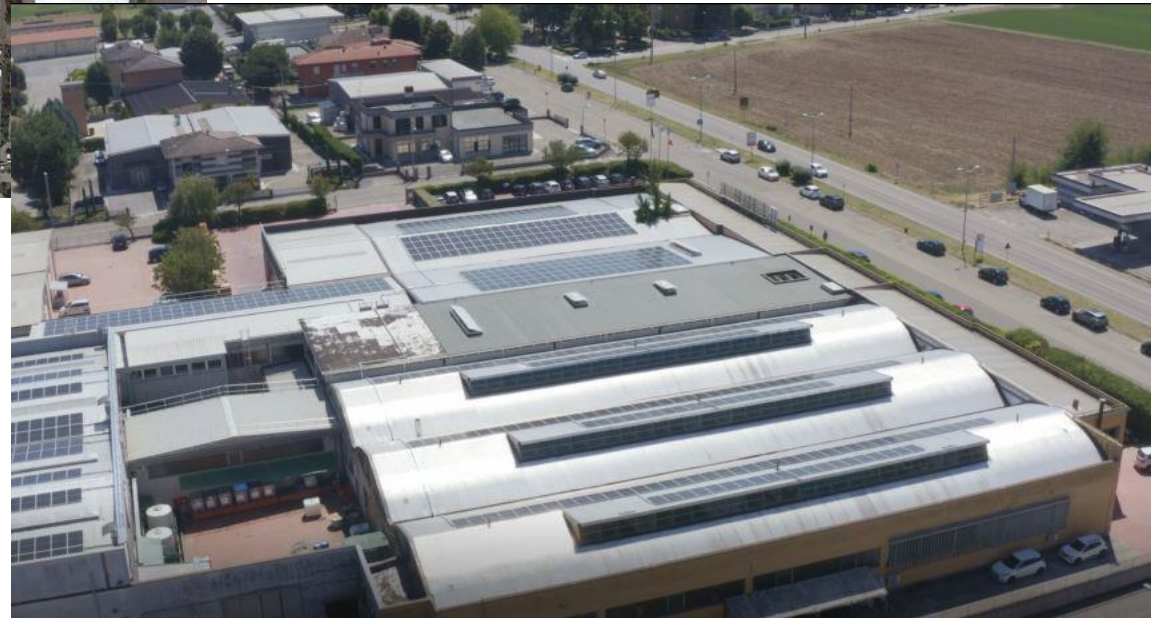
V. Fermi factory roof after photovoltaic plants installation
