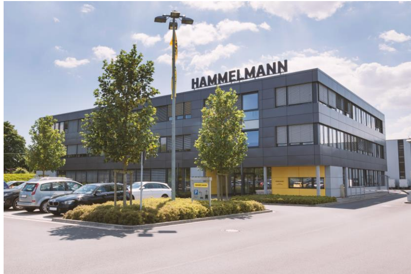
Hammelman, Germany – Oelde factory
