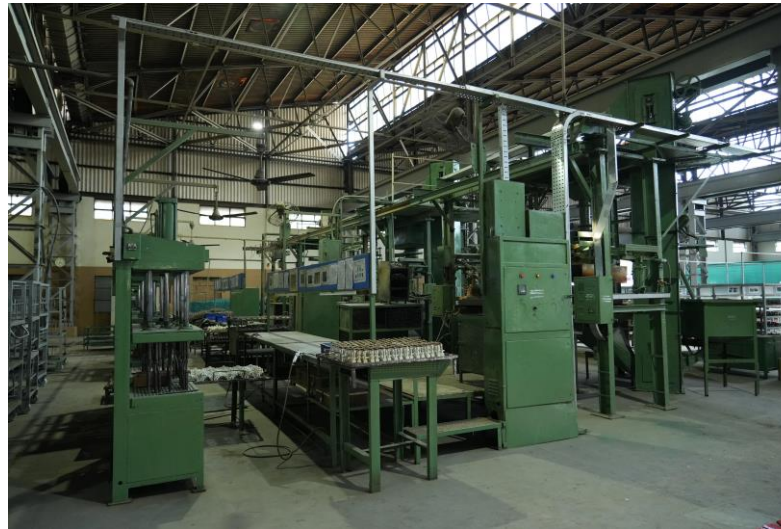
March 2023 – Indoshell factory after Group refurbishment
