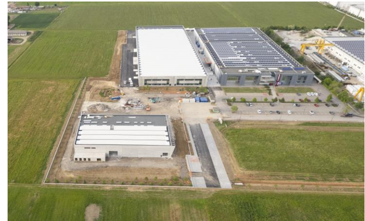
April 2023 - Cavriago new factory work in progress
