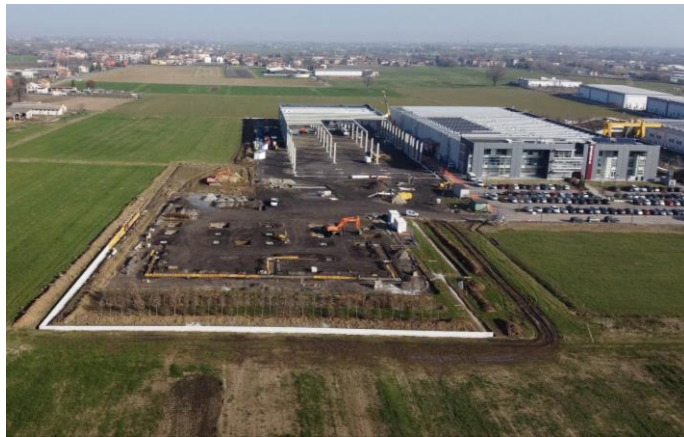
February 2023 - Cavriago new factory work in progress
